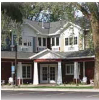
Gorecki Guest House, adding an additional 16 rooms to further benefit our patients.
